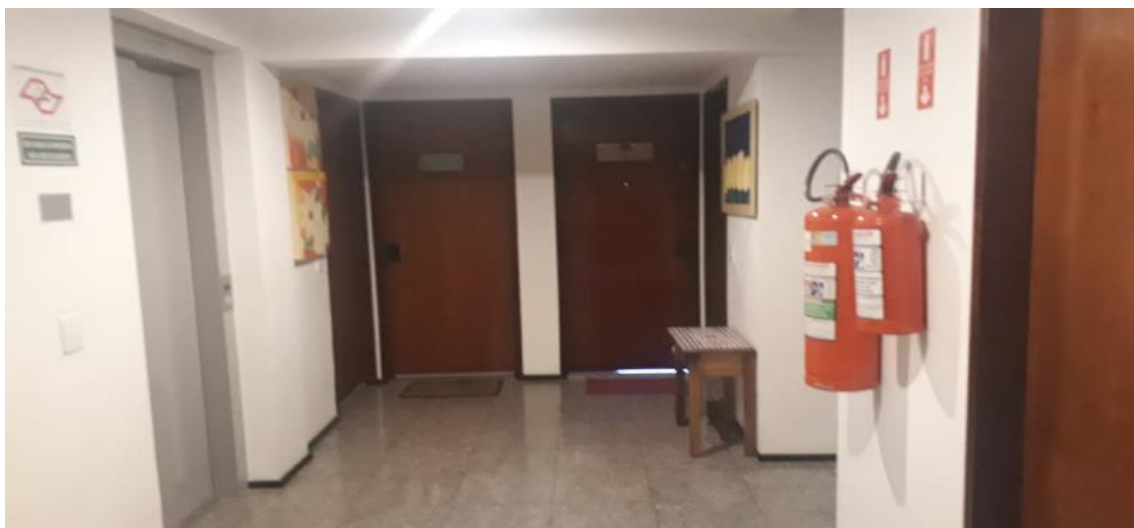
Hall do andar
