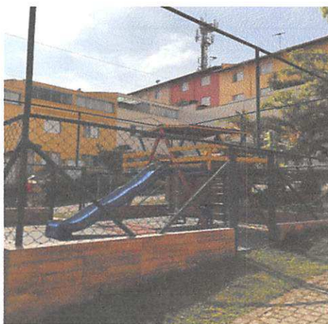
Vista do playground.
